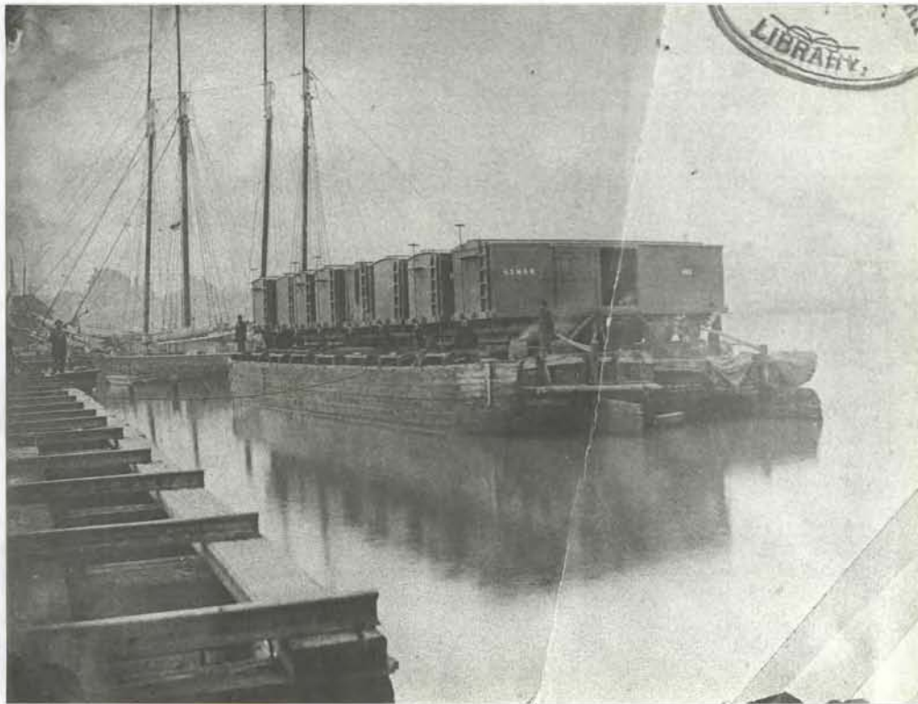
Plate 2. Canal Barges Carrying Rail Cars (illustration shows marine railway similar to Features 18 and 19)
